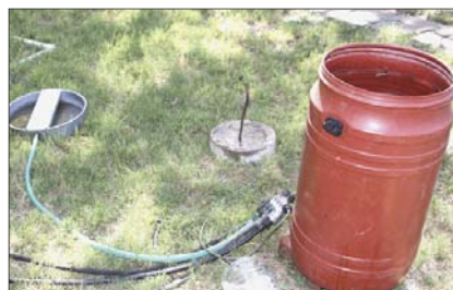
A simple 20-gallon rainwater collection tank feeds a birdbath, a pet waterer, and some landscape irrigation hoses at the historic Lowe House.
