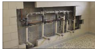
A wall is opened in the Clarendon Junior High bathroom to replace plumbing.
