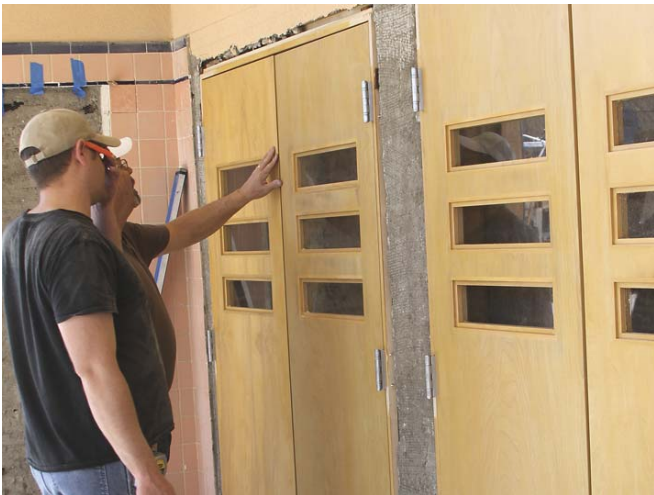
New look Contractors install new doors on the Mulkey Theatre Monday as part of the ongoing Phase One - Exterior Renovations to the 1946 building. The new doors were fashioned to match the design and stain of the originals. ENTERPRISE PHOTO / ROGER ESTLACK
