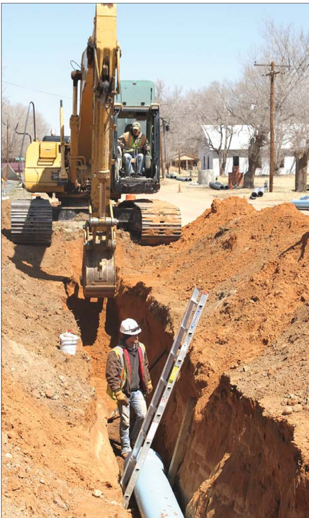
Workers install pipe for the Greenbelt groundwater project Monday on Sully Street in Clarendon.
