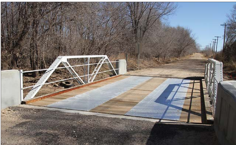
The Rosenfield Street Bridge opened for last week traffic following a half-million project that rehabilitated the structure and built a new bridge near City Park. The 1940 Warren truss bridge on Rosenfield was disassembled, reinforced, and rebuilt.
