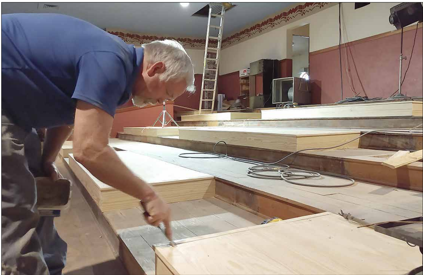
Leo Brewer with Pioneer General Contractors putties gaps in new decking in the balcony of the Mulkey Theatre Tuesday afternoon. The new decks will accommodate recliner seats that will be installed in the balcony next month.
