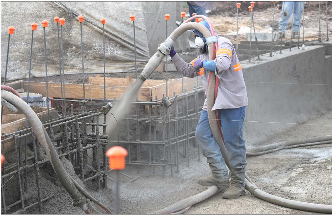
Progress! Workers sprayed gunite to form the walls of the new Clarendon Aquatics Center last Wednesday. The center is still on track to be finished and open this July, according to city officials.
