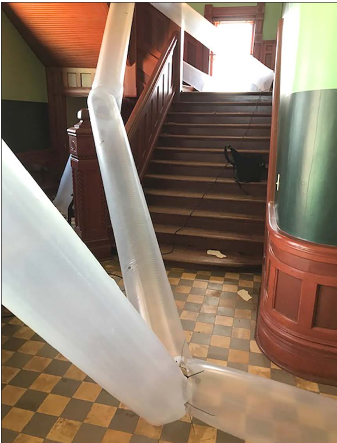
Turn up the heat Plastic ducting carries super-heated air through the Donley County Courthouse last week as workers continue to try to dry out the 1890 building after it suffered major water damage during the arctic storm last month.
