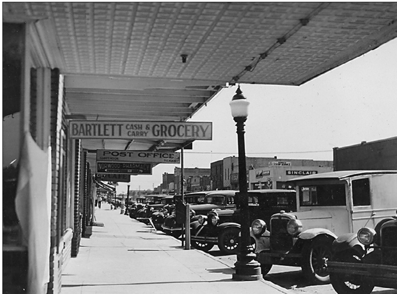
Ornamental street lights installed on Kearney Street in the 1920s were known as a "White Way" system. The term refers to a brilliantly lighted street or avenue especially in a city's business or theater district. Clarendon's White Way included 22 cast iron street lamp posts with 18 of those being along Kearney Street. A news article refers to the others being installed near the railroad, but other evidence points to one being installed on the Courthouse Square and another at the old City Hall. This image of Kearney Street in about 1930 is looking north from near Clarendon Insurance Agency's present location.
