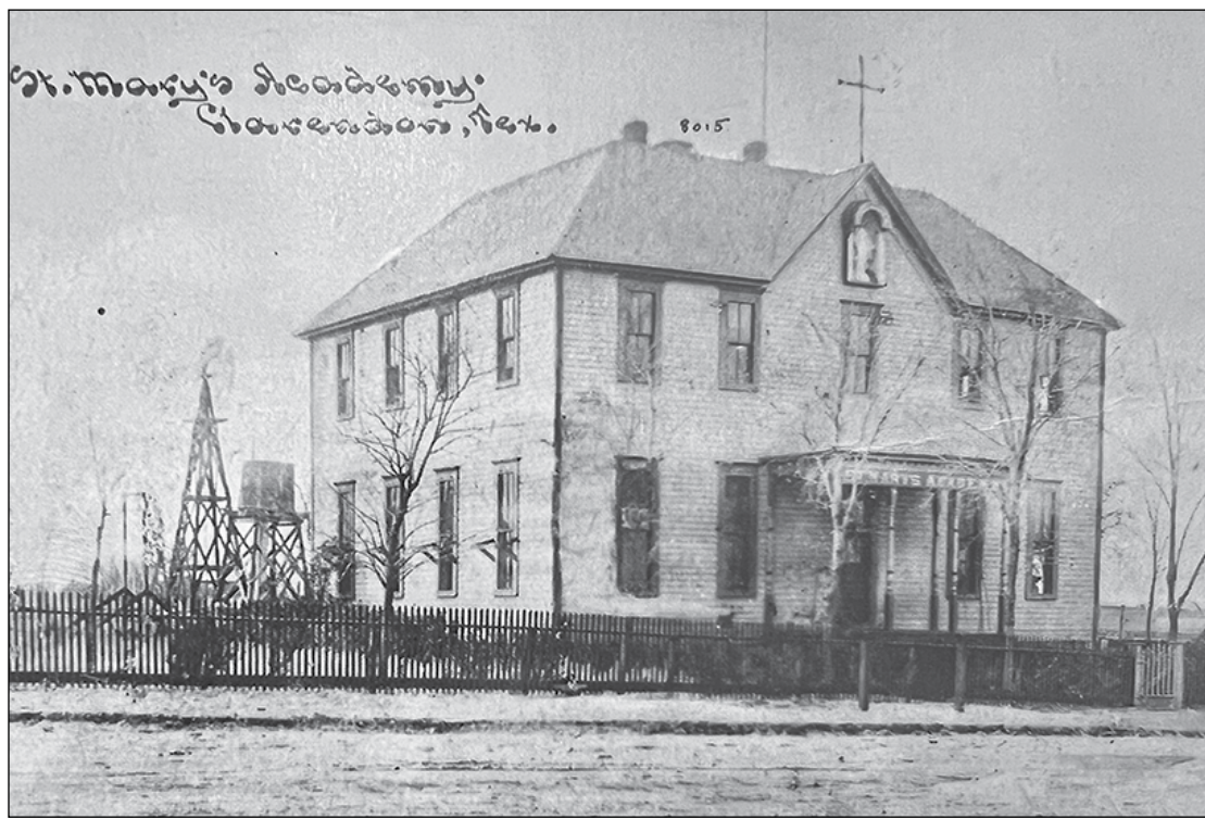
Saint Mary's Academy - about 1910: The Catholic academy opened in 1898 and stood on Montgomery Street between Goodnight and McClland streets before its closure in 1911 due to a typhoid epidemic. The building was later torn down and sold for lumber in 1918.
