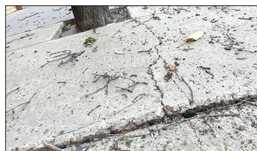
Trees were coming down at Herring Bank Monday as workers prepare for new sidewalks there as part of the Downtown Revitalization Project. The shallow roots of the trees had caused considerable damage to the old sidewalks, and the trees were removed to prevent similar damage from happening to the new sidewalks.
