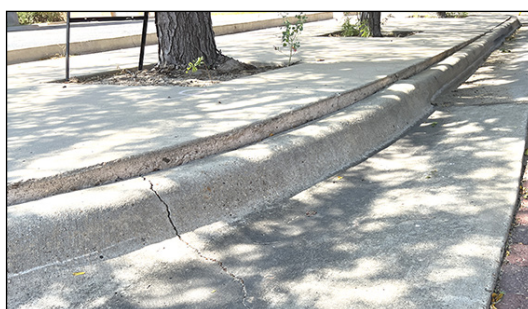
Trees were coming down at Herring Bank Monday as workers prepare for new sidewalks there as part of the Downtown Revitalization Project. The shallow roots of the trees had caused considerable damage to the old sidewalks, and the trees were removed to prevent similar damage from happening to the new sidewalks.
