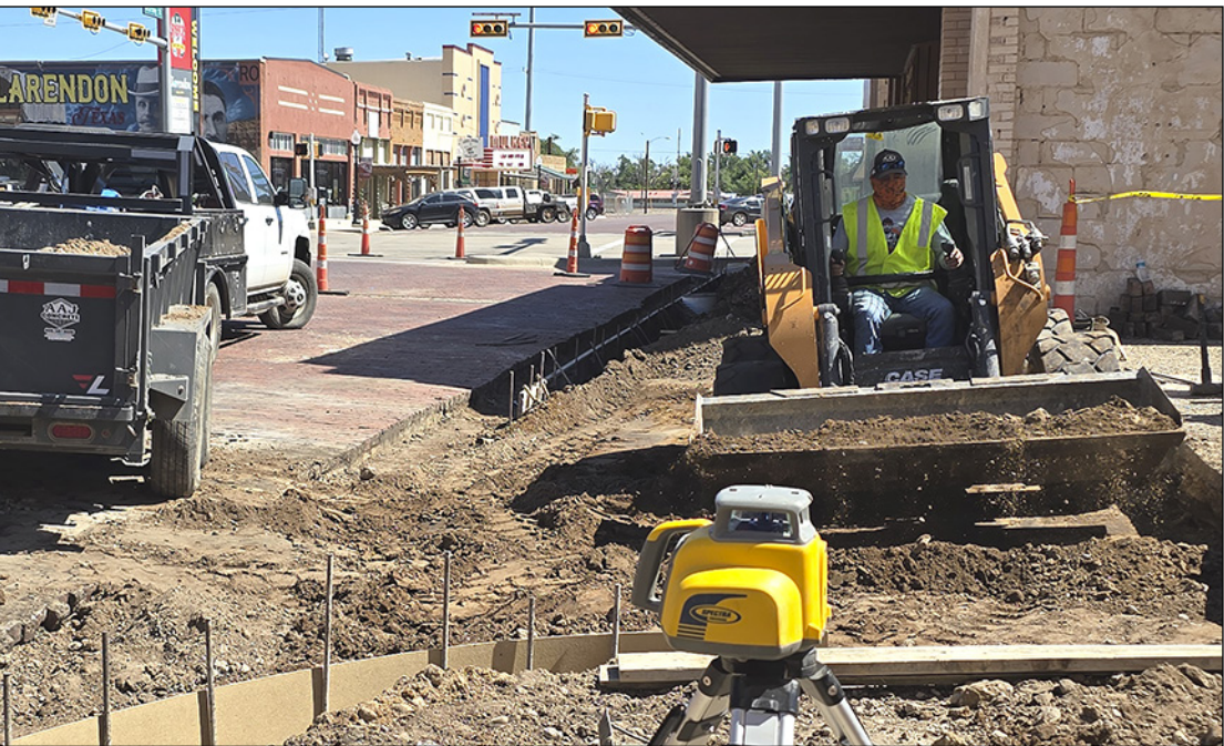
Phase 2 begins The second phase of Clarendon's Downtown Revitalization Project started in the 200 block of S. Kearney last week with sidewalk removal in front of the Donley County State Bank and the Masonic Lodge. Public Works Director said the contractor will start pour concrete this week for the new gutter as it continues to remove old sidewalks.
