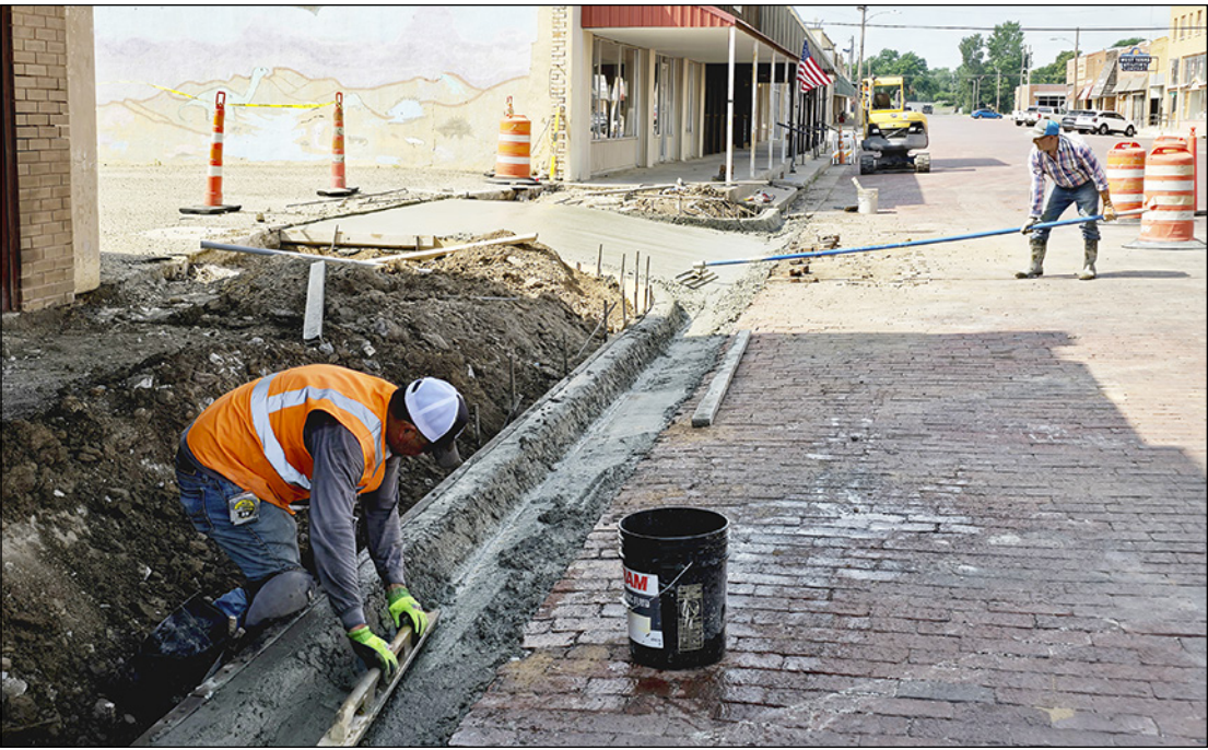
Progress Workers formed and began setting new curb and gutter in the 200 block of S. Kearney Street last week, starting in front of the Masonic Lodge. ENTERPRISE PHOTO
